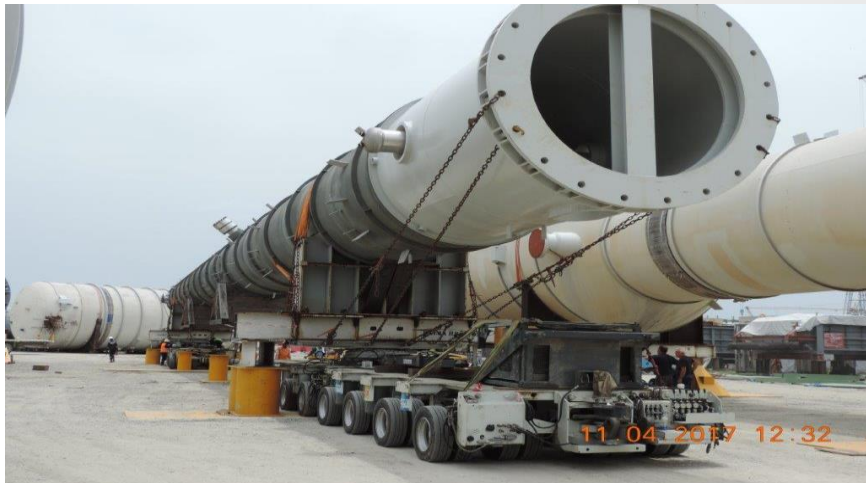
Urea reactor being offloaded at site
