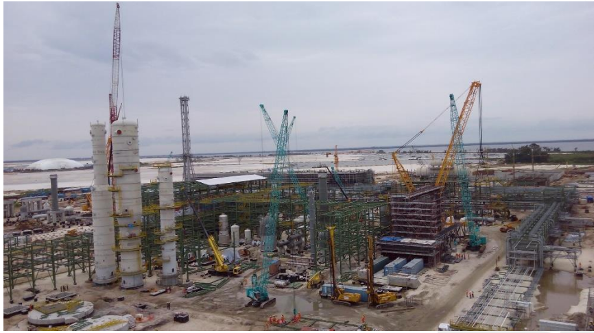
Pictorial view of the construction site
